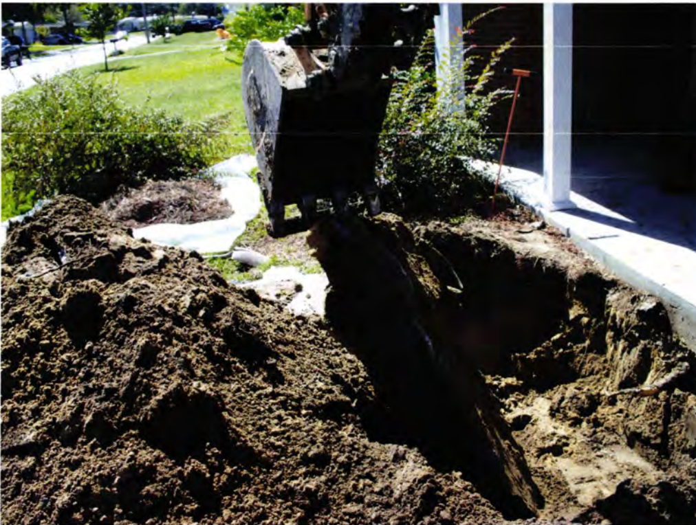
Picture 2: Concrete cap being removed from atop UST 326Ash.
